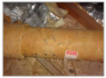
distributed heated air through rigid metal ducts which were wrapped in insulation. This was a big improvement over wall heaters found in most pre-1960 houses, but rigid ducts were difficult to install and were not sealed well.
