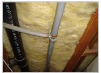
Unfortunately, many of these plumbing systems failed causing property damage. Although an exact cause could not be determined, it is expected that the chlorine in water caused the fittings to fail. In some early installations with aluminum crimps, the crimps failed due to thermal expansion. A huge class action lawsuit was settled with the manufacturers of the Polybutylene which paid to repair or replace plumbing systems which had failed.
