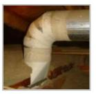
Determining the presence of asbestos is beyond the scope of a home inspection. But your home inspector should have the knowledge to recognize components that may contain asbestos. Replacing ducting that contains asbestos can incur added costs.
