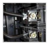
Aluminum wiring is still allowed on 30 and 40 AMP circuits which are used for electric ovens, AC condensers, clothes dryers, etc. These circuits usually are run directly from the panel to the appliance without any connections along the way and new connectors are compatible.
