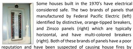
Some houses built in the 1970's have electrical panels that are no longer considered safe. The two brands of panels that should be replaced were
